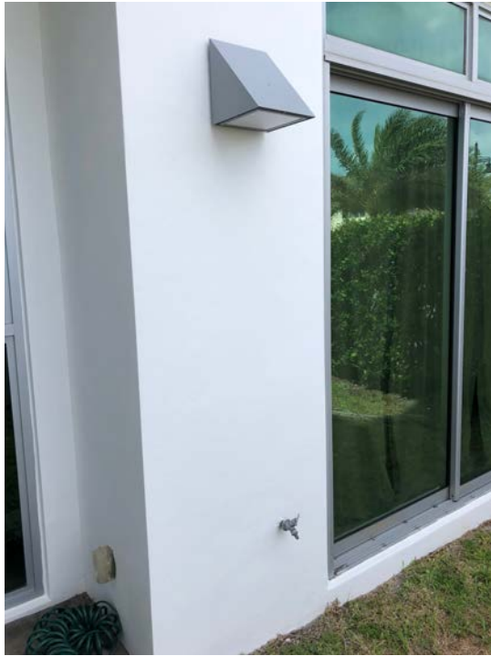
Examples of low maintenance shielded LED lighting
