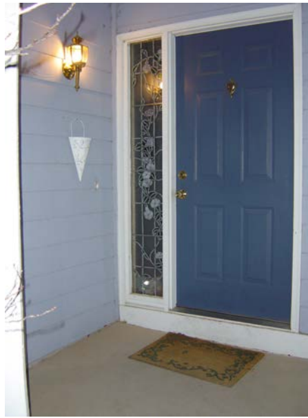
Examples of door vision panels on the opposite side of the door handle.
