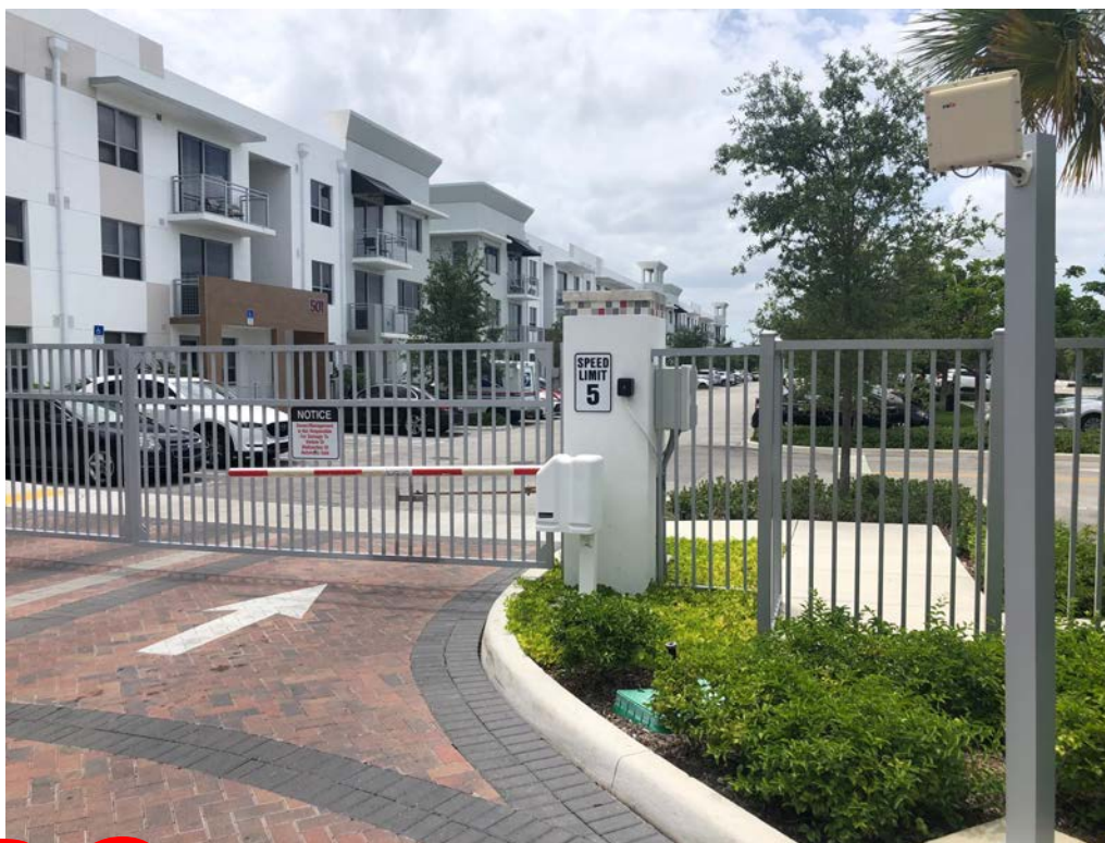
The reader on the right picks up the signals from decals or RFID stickers placed on residents' cars. The gate arm goes down after the car enters to stop tailgating.
