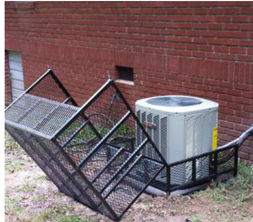
Examples of protecting the AC compressors on ground level.
