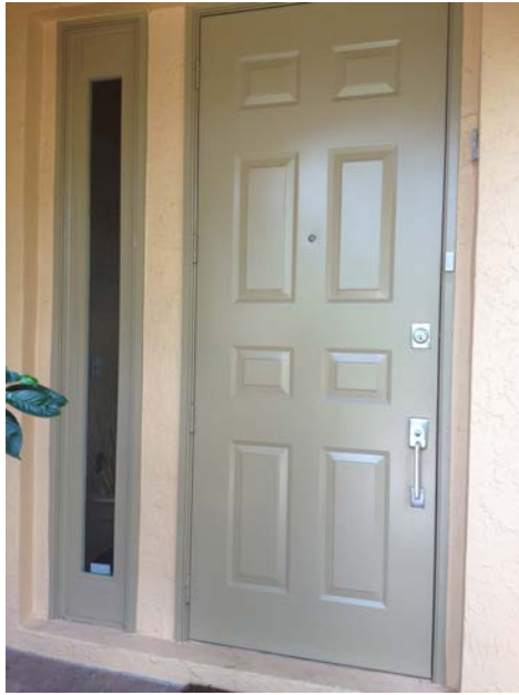
Examples of door vision panels on the opposite side of the door handle.
